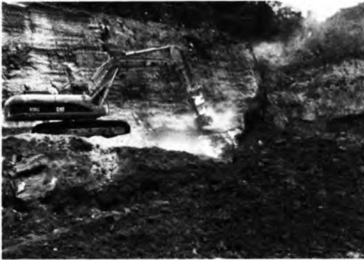
Photo 2: A view of mounted twin cutter in operation.
